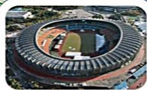
Seoul Olympic Main Stadium
